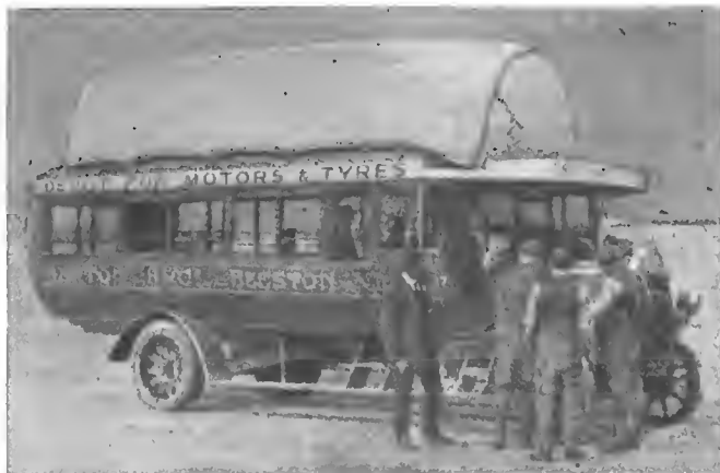
English bus equipped for running on uncompressed town gas
